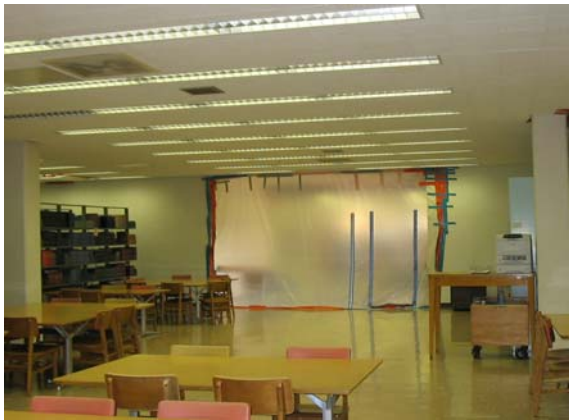
Second floor up to the addition was open and they were getting ready to open the rest of the second floor when this picture was taken. Plastic cover between the two sections was still in place.
