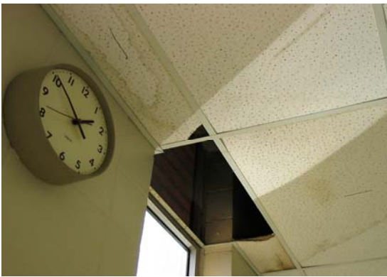
Library third floor addition near north wall
